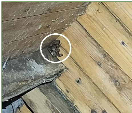
Plate 3.14 –Brown Long-eared Bats roosting in S02 on internal inspection.
