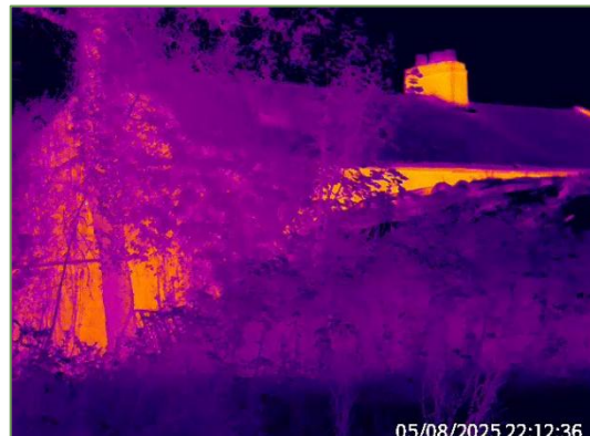
Plate 3.15 – Thermal camera coverage of S04.
